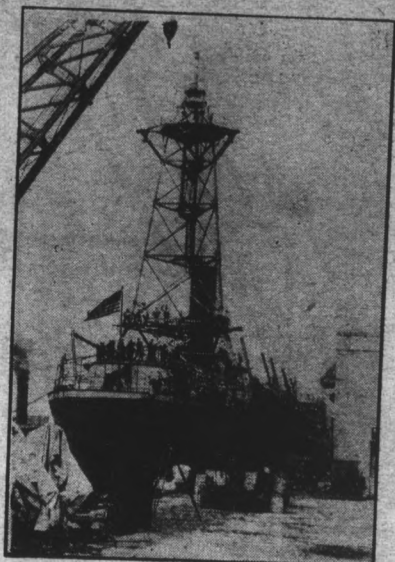
The S. S. Patoka is the first U. S. vessel to be equipped with mooring masts for dirigibles.
