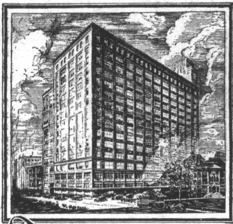
The New 15 Story Building (Now Under Construction)
