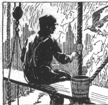
This painter is risking his life to give the steel cables of the Brooklyn Bridge paint protection. He is putting on red-lead, the strongest shield that steel can have against rust.
