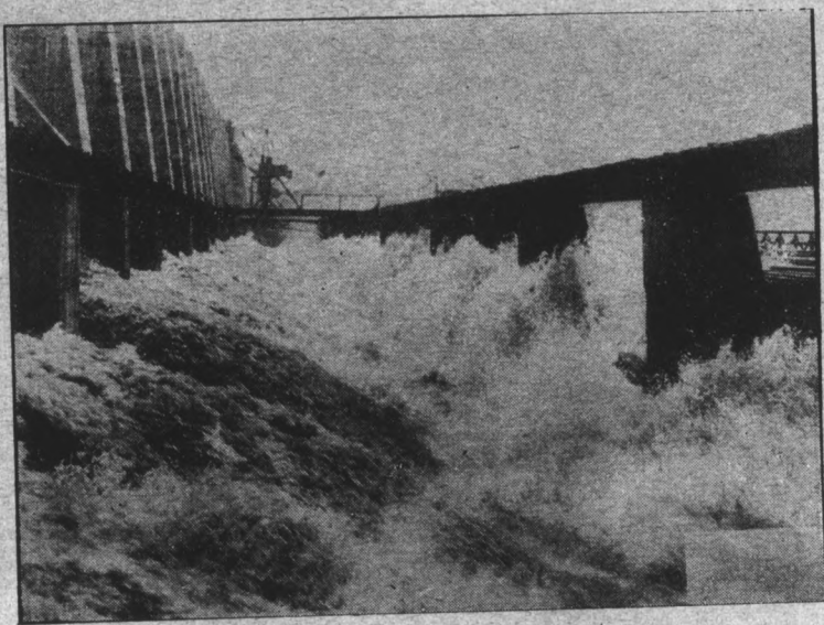
The Muscle Shoals power project nears completion as the Wilson dam begins to function. There is a deafening roar and splash as this spillway section discharges through Coffey No. 2.
