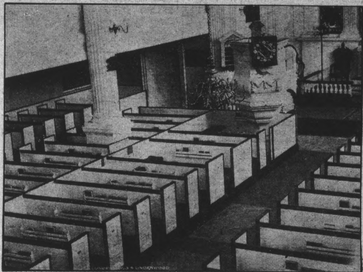
Old Christ Church, Philadelphia, has recently been equipped with a modern sprinkler system to protect it from fire. Here Washington, Adams, Franklin, Penn and Betsy Ross worshiped.
