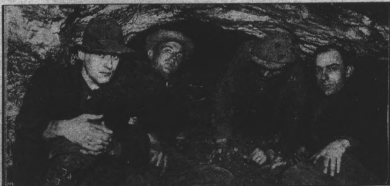
These four men are far beneath the Hudson River in a tunnel which will be used for automobile traffic between New York and New Jersey. This picture shows where the borings meet.
