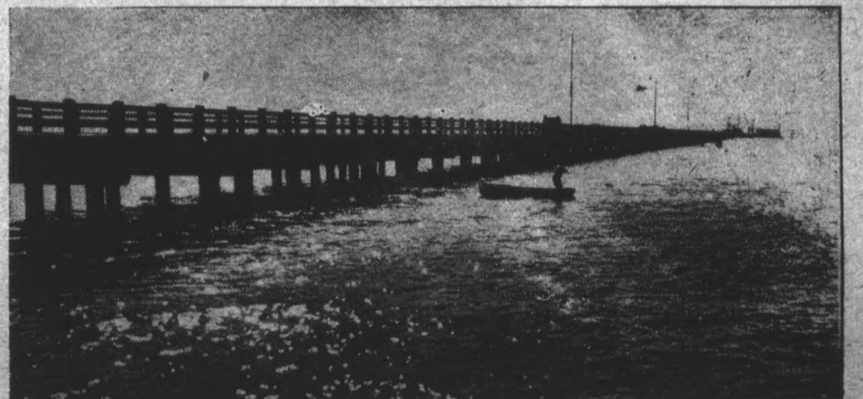
The Gandy Bridge, spanning Old Tampa Bay and connecting Tampa and St. Petersburg, Florida, has just been completed. This great concrete structure is the longest auto toll bridge in world.
