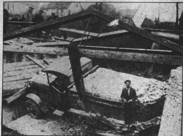
Because this man did not believe in signs he drove a six and a half ton truck loaded with eight tons of brick on a five-ton bridge. This was the result.
