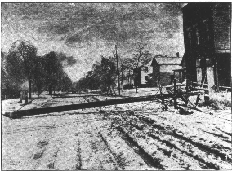
The recent sleet storm tore down cables and poles in Springfield, Illinois, and did damage to the amount of four million dollars within a radius of forty miles.
