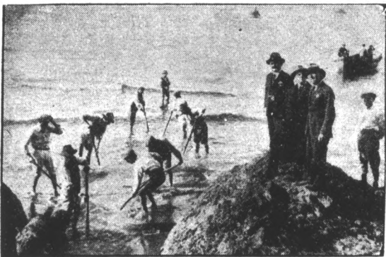
Landing at Anzio, Italy, the European end of the first direct Italy-U. S. cable, which will connect directly with Rome.
