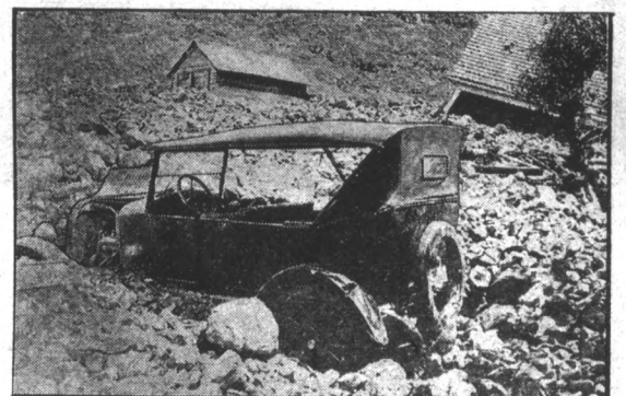
Great damage was done by combined electric and hail storm at Asotin, Idaho. The Asotin Creek carried the refuse shown here.
