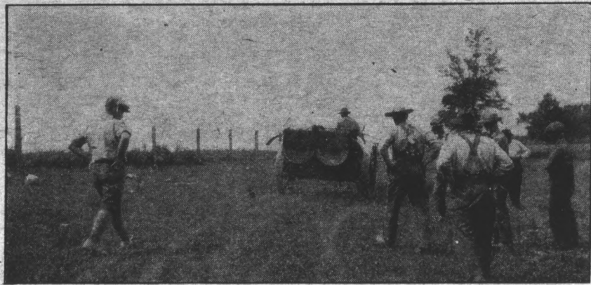
The Marl Was Spread Rapidly With an Ordinary Manure Spreader.
