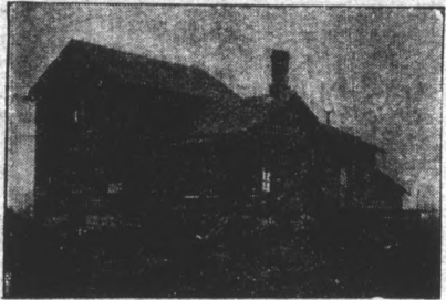
This House, Failing to Keep up with the Times, Drove its Occupants to Other Quarters.
