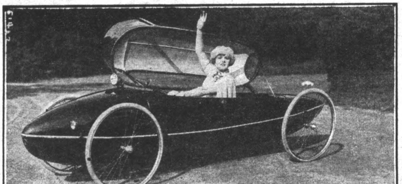
"Landskiff" is a hand-propelled machine, weighing forty pounds and capable of attaining a speed of thirty-five miles an hour. It was invented by Dr. Manfred Curry, of New York.
