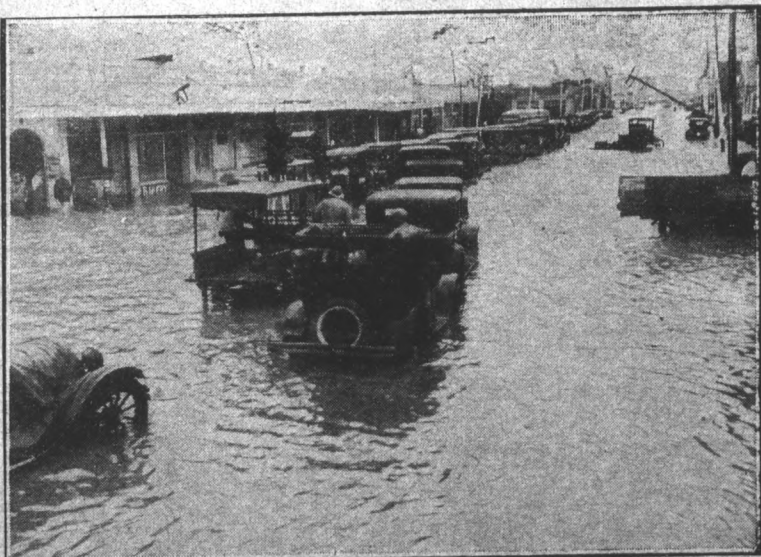
Autos were abandoned in the street when caught in the flood which accompanied Miami's hurricane. The rushing water put the generators and motors out of commission.
