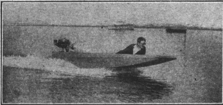
This motor boat, built by Dr. R. F. Fiske, who spent only $12 in the building, broke an unofficial world's record by making 23.11 miles an hour.
