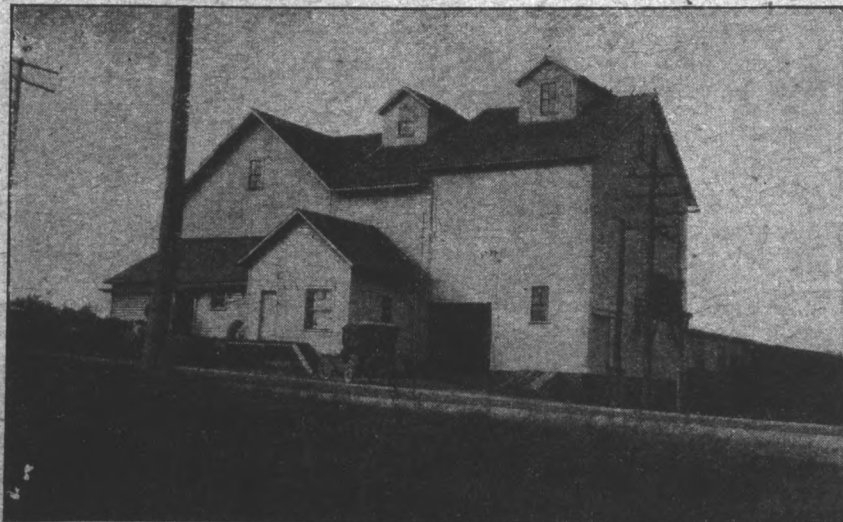
Elevators Are Usually Made of Steel to Cut Down Fire Hazards.
