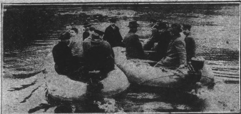
An ingenious German inventor has devised this collapsible life boat which, when deflated, can be carried about as an ordinary piece of luggage.
