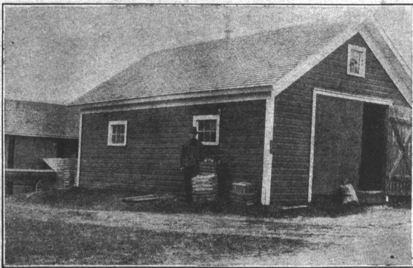
Mr. Lincoln and His Very Efficient Storage Building, which is Equipped with Underground Duct and Ventilator Systems.
