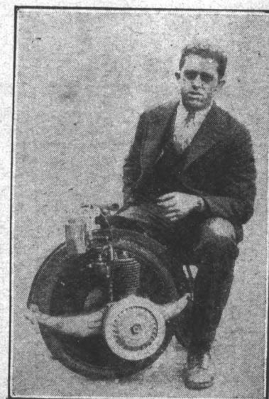
The rider's feet are the only brakes on this motorcyclette invented by William Nichols.
