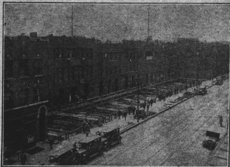
A 350-foot front in Chicago is being moved by screw jacks. When the foreman on the job blows the whistle, each man at the screw jacks makes a turn which moves the frontage evenly.
