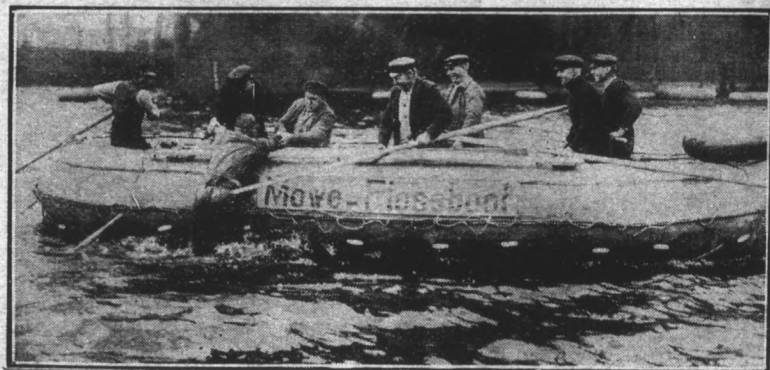
A rubber life boat which is collapsible, and capable of carrying a load of sixty persons, proved successful on the first try-out. The boat can be inflated in twenty minutes.
