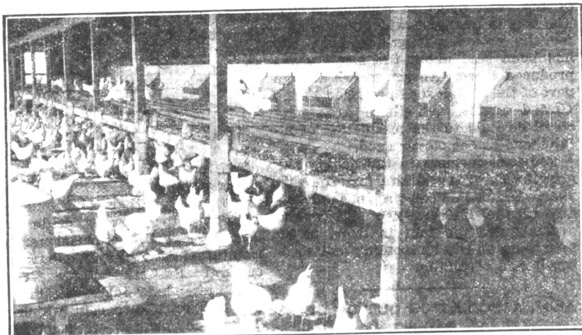
The Dropping Board in this House is Located Six Feet from the Back, with Nests on the Rear Wall.
