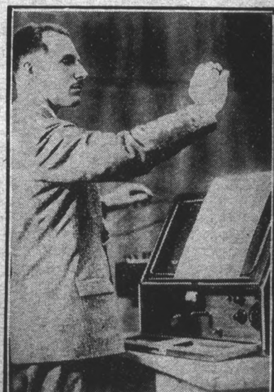
By motion of hand over this ether wave instrument, music is produced.
