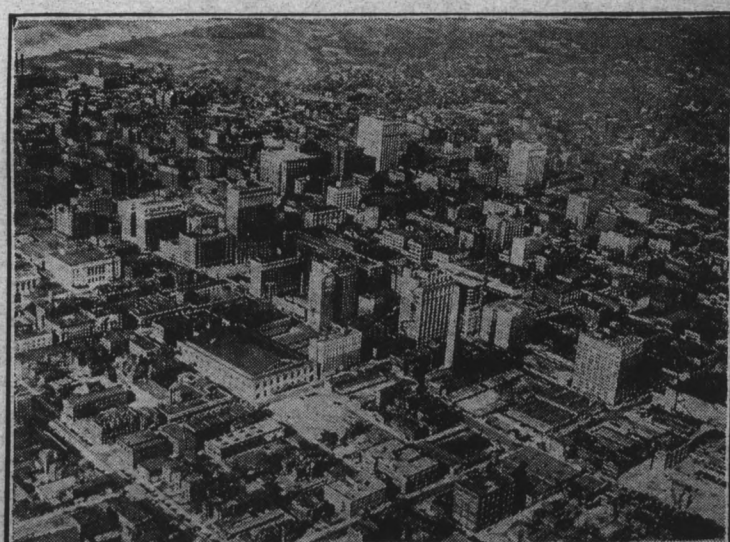
An airview of the business section of Kansas City. The low white building with the wide roof is the Convention Hall where the Republican Convention will open June 12.
