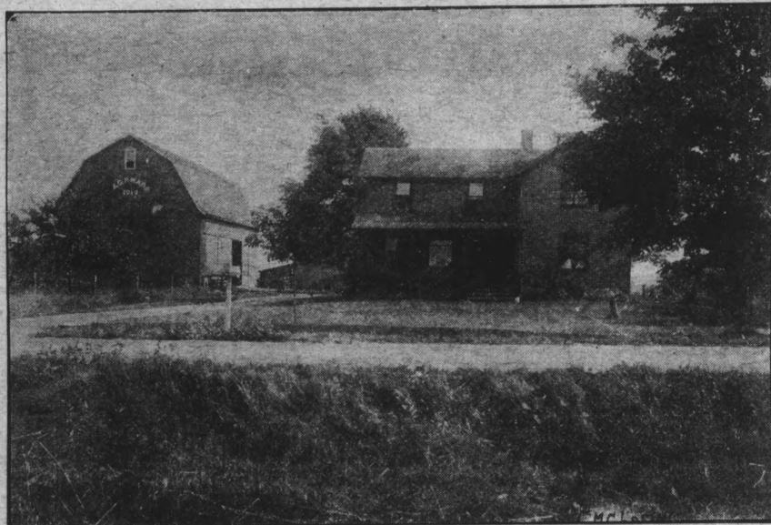
Good Lights Plus an Ever-Ready Source of Power, That Costs Little, Yield Worth While Profits and an Abundance of Satisfaction
