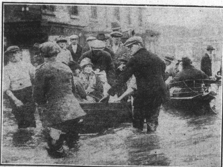
History is reversed and the waves rule Britannia. This deluge in London, England, caused by abnormal tides flowing in from the North Sea, resulted in millions of dollars property damage.
