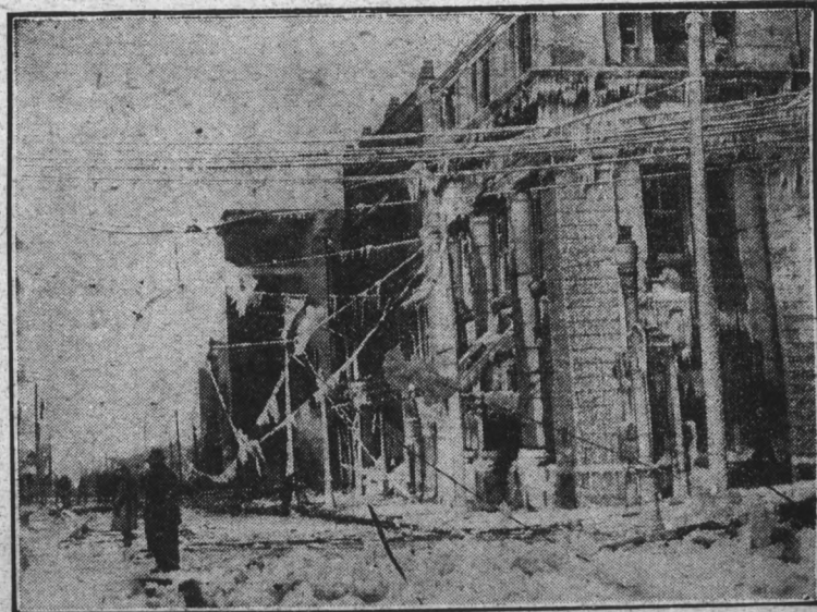
For the second time in twelve years, a large section of the business district in Fall River, Massachusetts was destroyed by fire. The damages are estimated to be $20,000,000.
