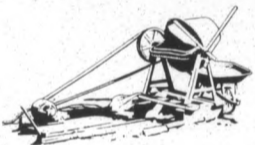
An electric motor takes the heavy labor out of concrete mixing.
