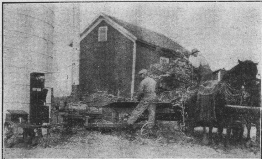
With the Electric Motor Attached Directly to the Cutter Frame, it Was Possible to Do This Work Economically with a Small Crew
