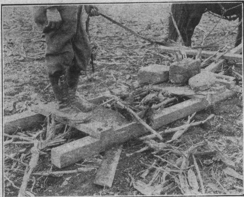
This Home-Made Outfit Was Designed to Cut Corn Stubbles Down to the Ground and Is Useful in Fighting the Corn Borer
