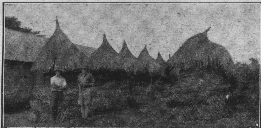
African Corn Cribs Made of Baked Mud and Vermin Proof Coverings
