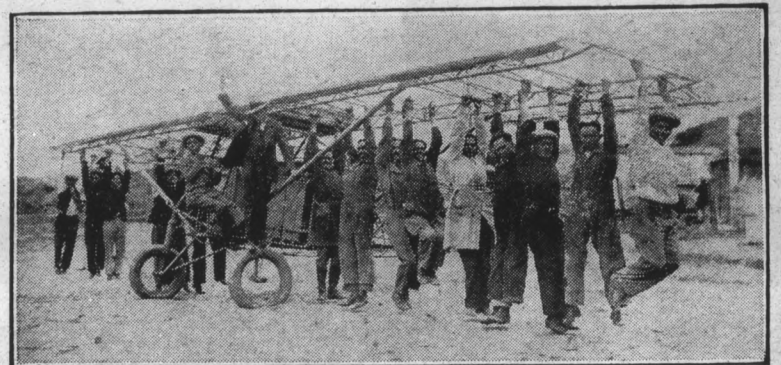
Eighteen men, hanging and pulling on the framework of the Mexican Army's first all-metal plane, did not break or bend it although their combined weight blew a tire.
