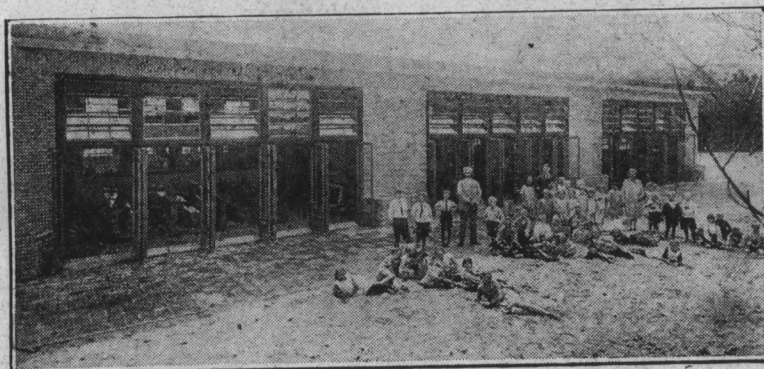
One of the new school houses being built in Amsterdam. Instead of stuffy classrooms, the building consists of a roof—for rain—and doors and windows to insure fresh air all the time.
