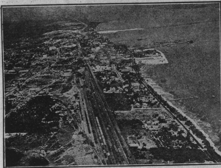
An airview of the city of Fort Pierce which was damaged to the extent of more than one million dollars by the hurricane that swept Florida's east coast recently.
