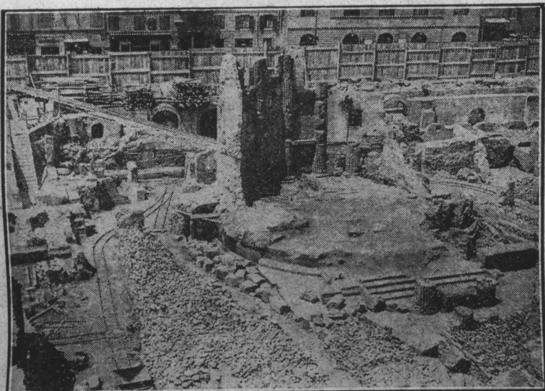
The ruins of a mediaeval temple was discovered by workmen who were excavating for the erection of a new theatre in Rome, Italy. Notice the well preserved walls of the old temple.
