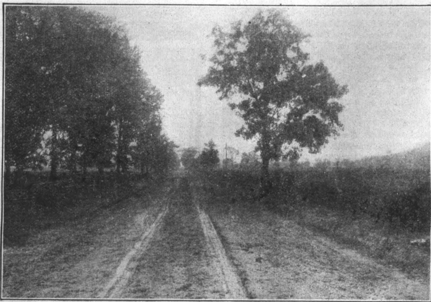
A Country Road Graded for Graveling According to Specifications for State Reward.
