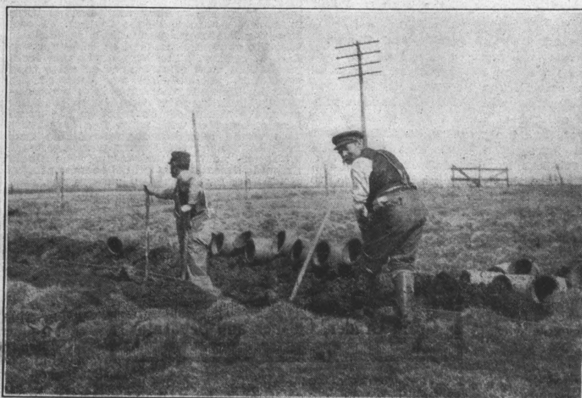
Laying Tile Drains in Swamp Land. (See Reclaiming Waste Land.)
