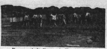
Busy asphalt-diggers in Trinidad Lake
