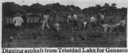
Digging asphalt from Trinidad Lake for Genasco
