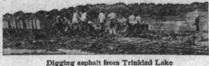
Digging asphalt from Trinidad Lake
