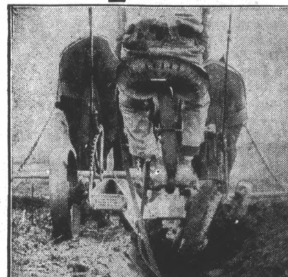
From Actual Photograph Spalding Deep Tilling Machine preparing a 12 to 16 inches deep, level, mellow, moisture-retaining seedbed, all in one operation.
