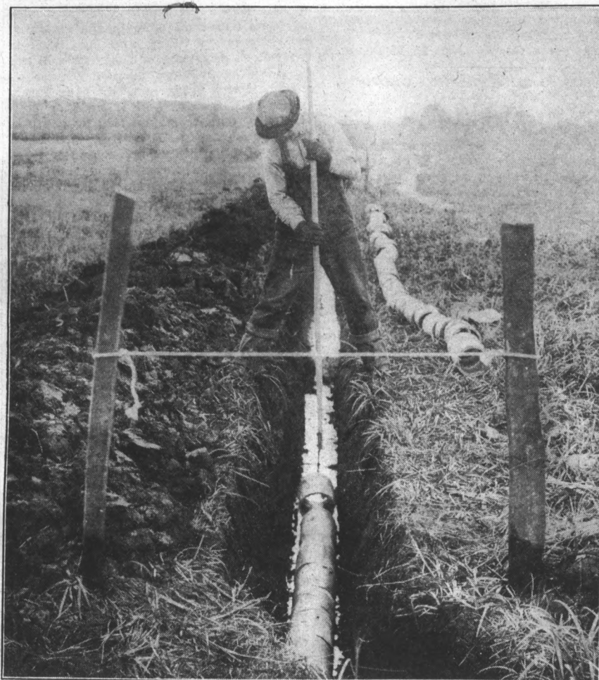
Laying Drain Tile with a Tile Hook.
