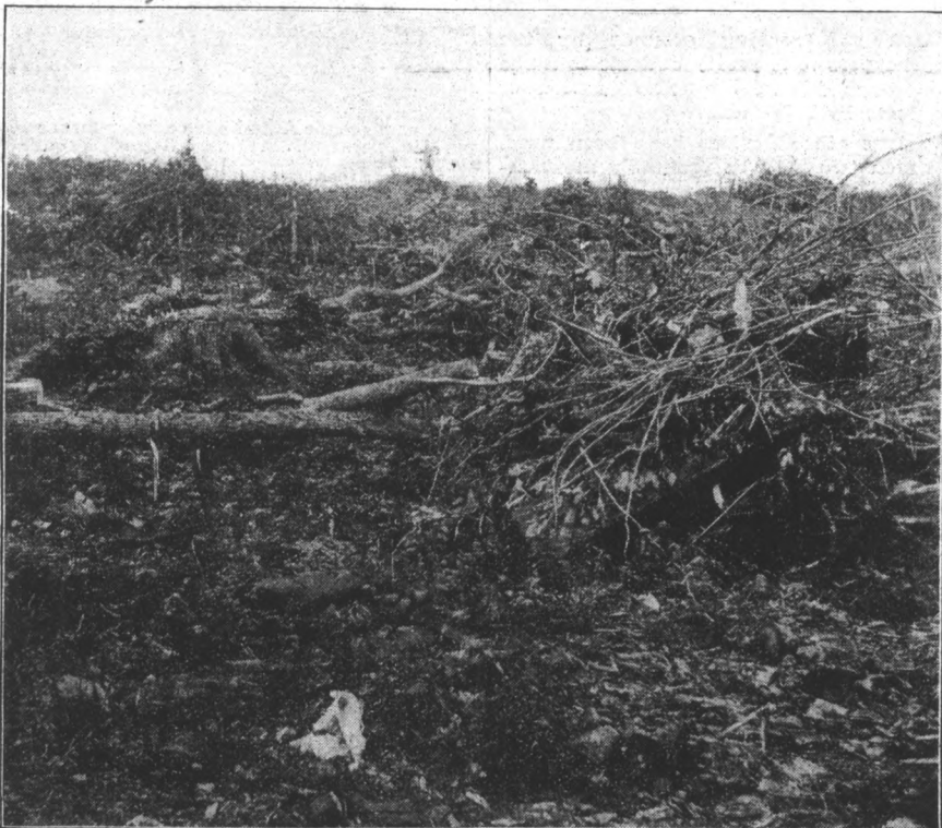
Fig. 2. Snags Pulled and Piled with Brush and Refuse Ready for Burning.
