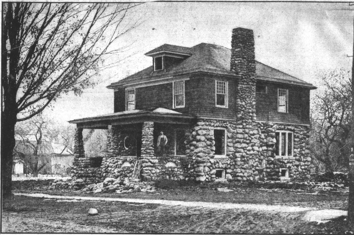
A Type of Field Stone Construction Popular in Sections where the Material is Plentiful.
