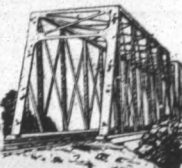
Built Like a Steel Bridge
