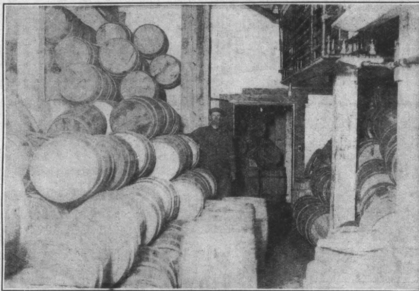
Apples Stored in a Large Farm Cold Storage Plant with Chemical Pipes Showing Overhead. (See page 502).
