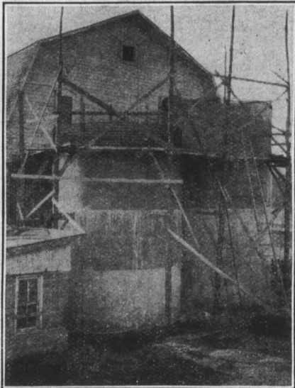
Steel Cored Silo in Process of Construction.
