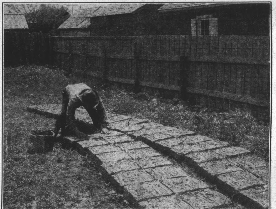
Placing Adobe Bricks in the Sun to Bake.
