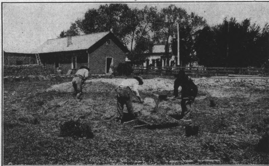
Mixing Adobe Preparatory to Making into Bricks.
