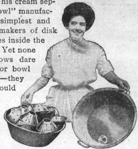
One pan contains the single little piece used in Sharples Dairy Tubular bowls. The other contains nothing but disks from a single "bucket bowl." Which is simple and easy to clean?
