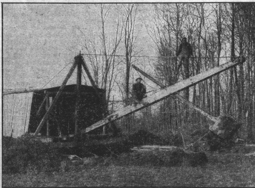
Type of Dredge Used in Digging Open Ditches to Provide Outlet for Tile Drain.
