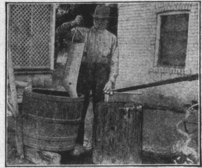
Showing a Farmer sharpening and re-tempering his ACME Share at home.
