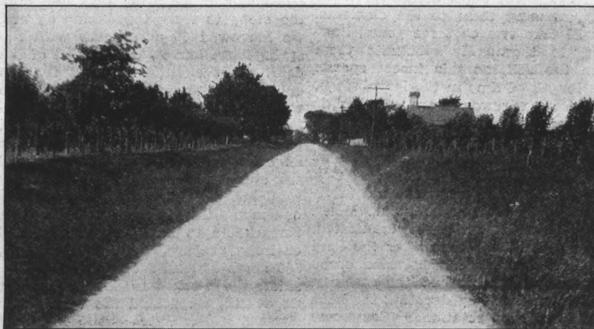
A "Ribbon of Stone" Typical of Permanent Roads Built in Berrien Co.
